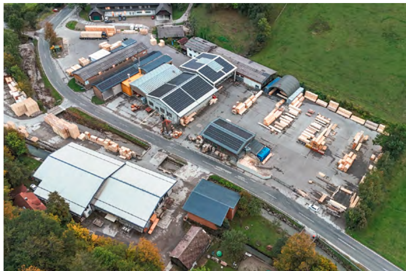
Use of self-generated solar power at the Ramsau site (Austria)
